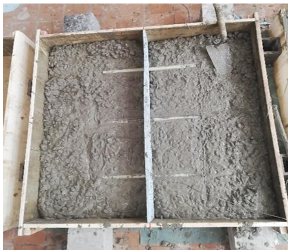
b) Complete mold with dowels.
